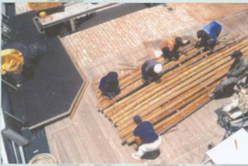
Bamboo poles are tied tightly with the iron frame
