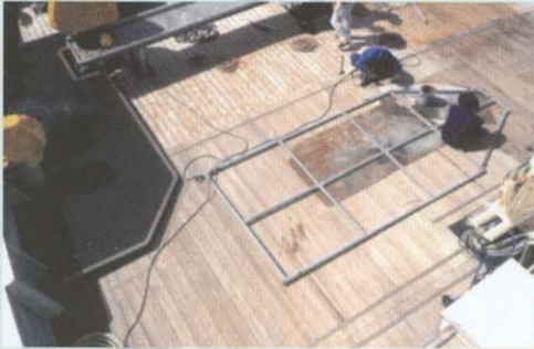
Structuring the iron pipe frame
